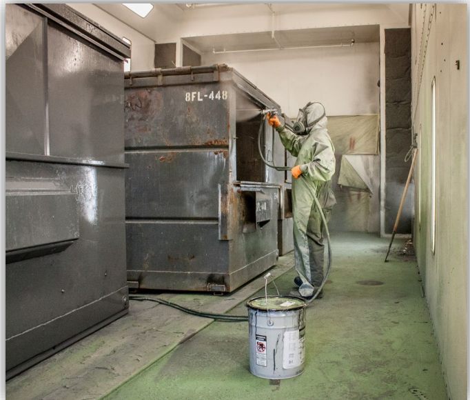
CWD employee refurbishing an 8-yard front load can
