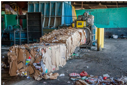
Paper being baled through CWD's baler
