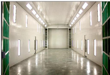
CWD on-site container paint facility
