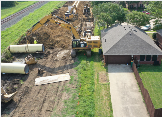
Our team coordinated with nearby homeowners to facilitate construction during our Parallel Pipeline project.
