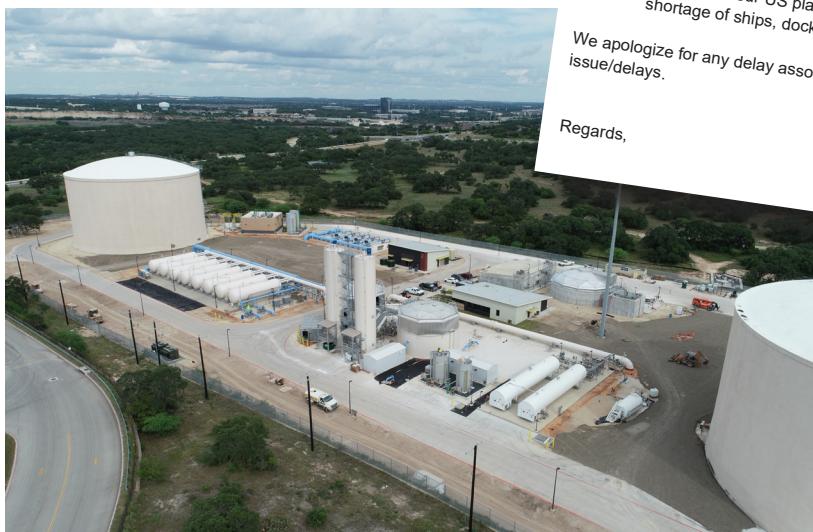
SAWS Agua Vista Station Completed on-time during the COVID Lock-down
