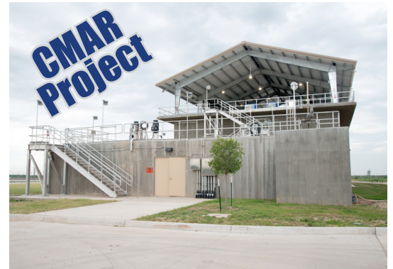
Hamby Wastewater Treatment Plant Award winning project completed on-budget
